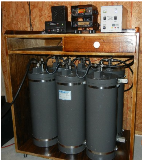
146.90 MHz Repeater Activated Sep. 10, 2019
