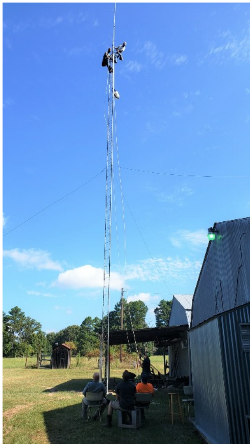
146.90 MHz Upshur County Repeater Antenna August 17, 2019
