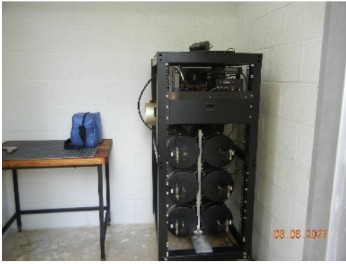
Repeater mounted in building.
